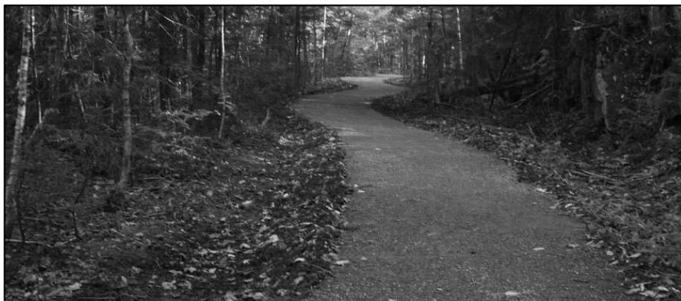
Completed ADA trail built by Hermit Woods Trailbuilders, LLC in Worcester, VT
