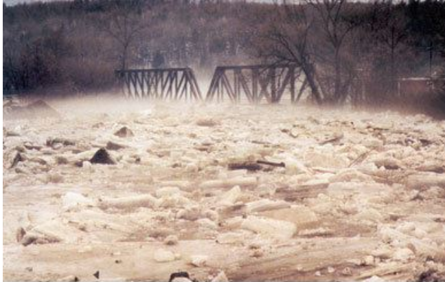
Figure 3: A view of the ice and the still intact railroad bridge from the Taylor Street Bridge. Source: https://www.montpelier-vt.org/604/Flood-of-1992
