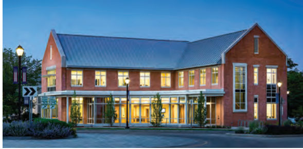
Town of Middlebury Town Offices
