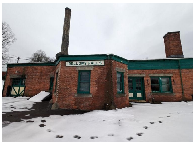
Bellows Falls Train Station building, March 2024. The station is being transformed into a multi-modal transportation hub after historic preservation, flood protection, and remedial actions. CAP implementation was completed under Stone's oversight.
