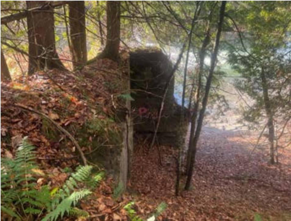
Photo 5. View of Hidden Dam retaining wall, facing south.
