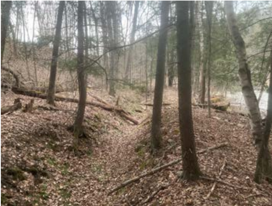
Figure 17. View of CDFC Upper Dam Penstock Trench outside of the Study Area.
