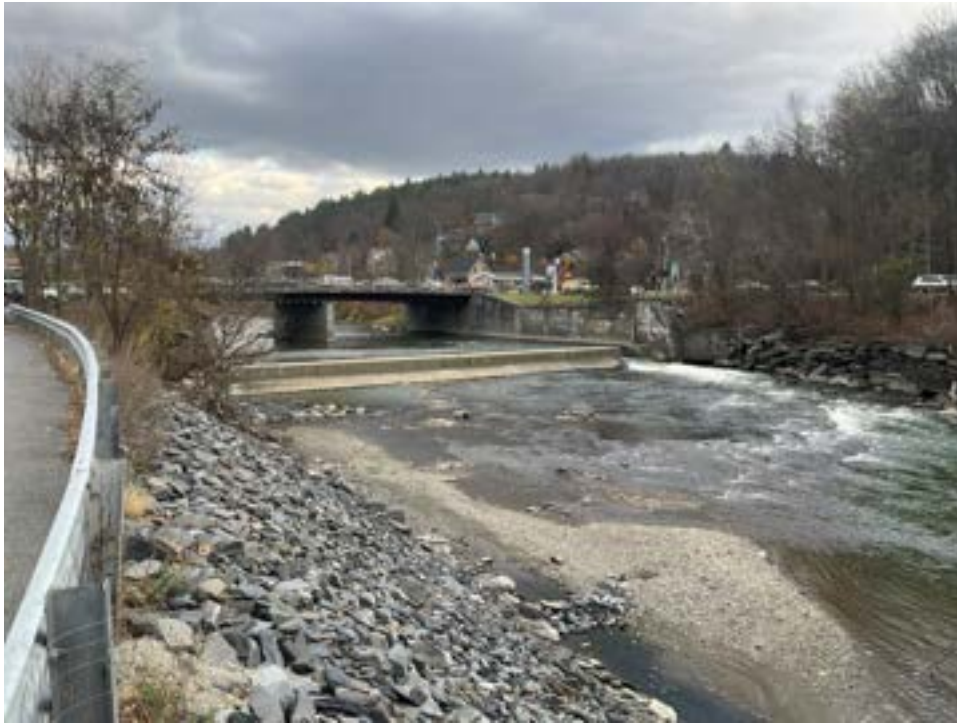
Photo 38. View of the Bailey Dam, facing southwest.
