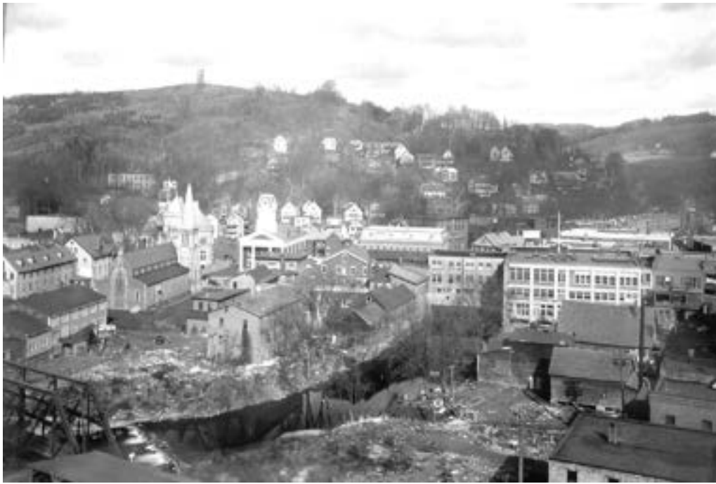
Figure 6. c.1925 Photo Depicting Trestle Dam at lower left (Photo Courtesy of the Vermont Historical Society).
