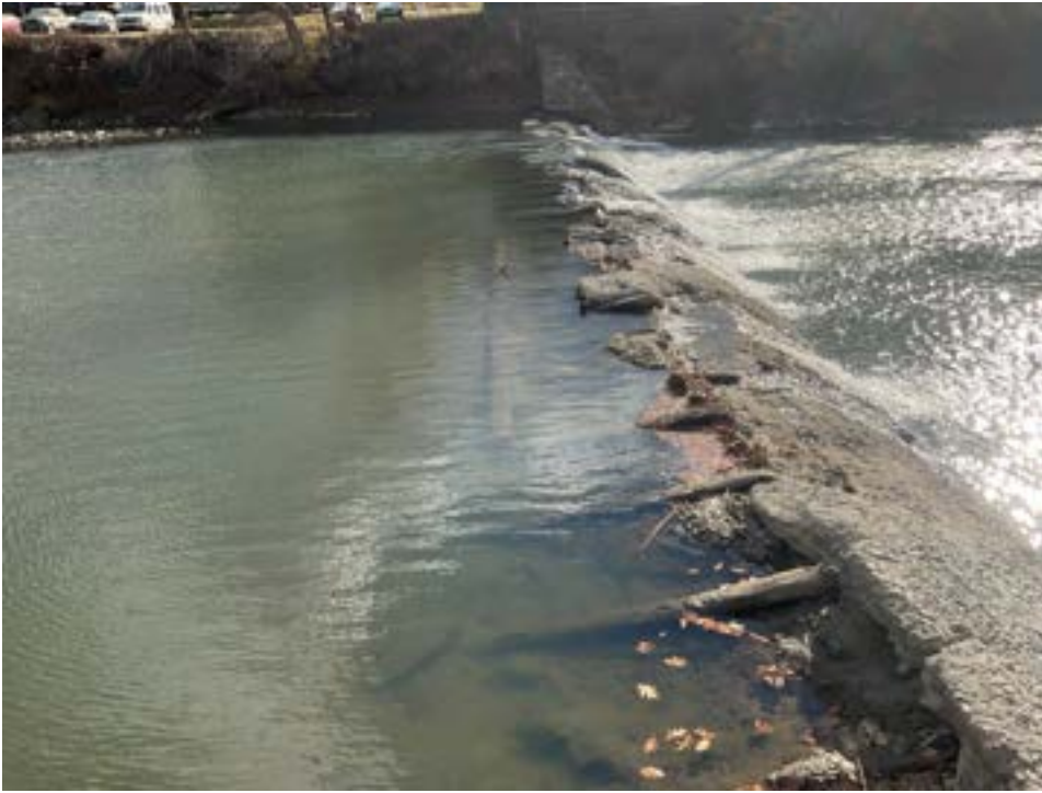
Photo 28. View of Pioneer Dam timber crib and concrete dam elements from north bank of the Winooski
