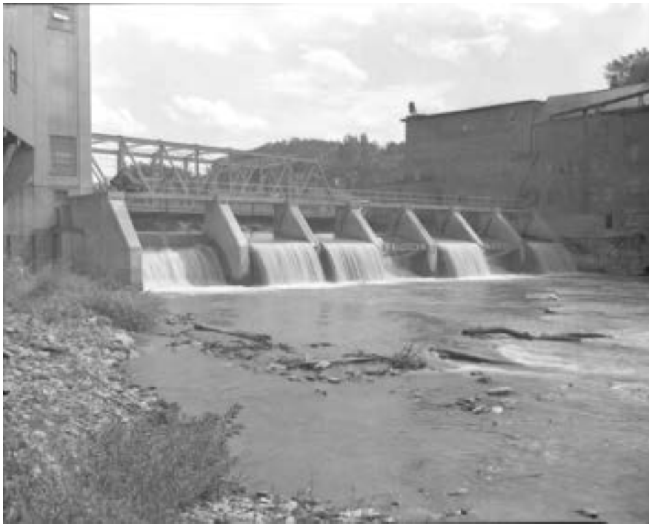
Figure 5. Photo of the Bailey Dam reconstructed in 1934, unknown date. Note the Berlin Mills and facilities associated with the E.W. Bailey Grist Mill are visible (Photo Courtesy of the VRC).
