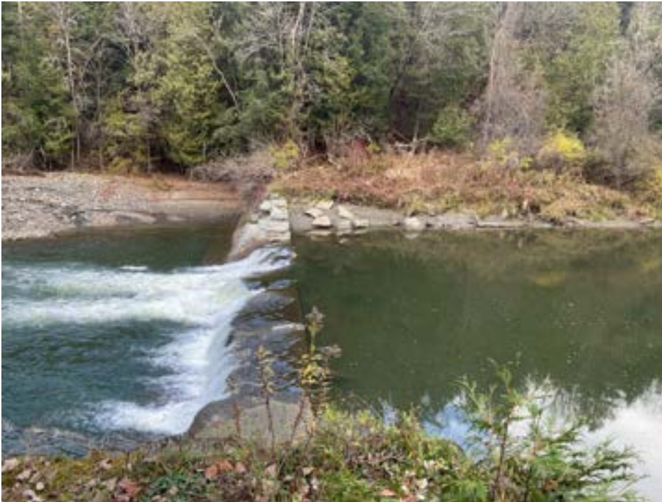
Photo 8. View of Hidden Dam from south bank of the Winooski, facing north.
