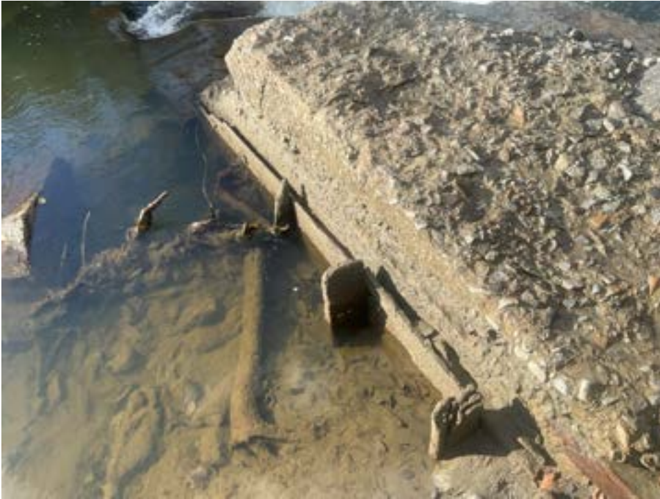
Photo 6. View of fragmentary timber dam elements at the Hidden Dam along the north bank of the Winooski River.
