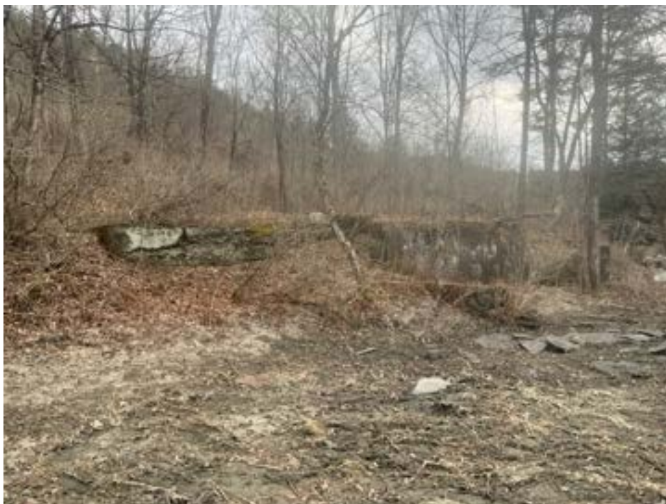
Figure 16. CDFC Upper Dam Powerhouse Foundations Remains located outside the Study Area.
