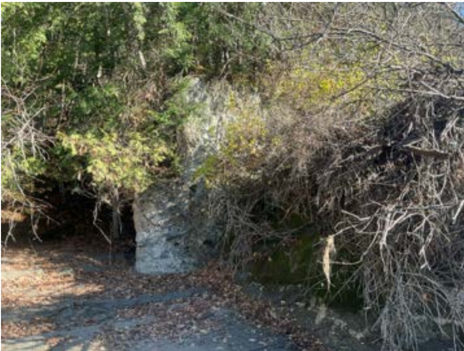
Photo 7. View of structural Hidden Dam elements from the north bank of the Winooski, facing north.
