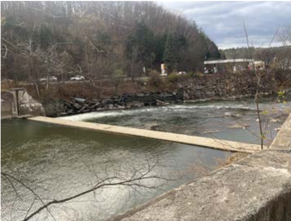
Photo 41. View of the Bailey Dam and stone embankment walls from the former Pioneer Mills, facing northwest.
