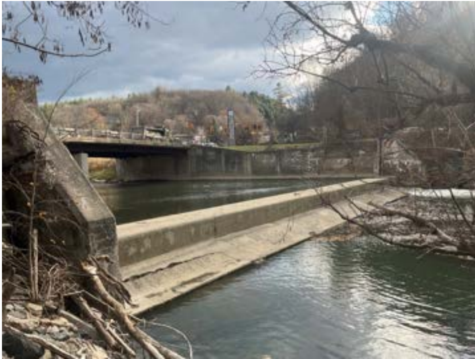
Photo 39. View of the Bailey Dam, facing southwest.
