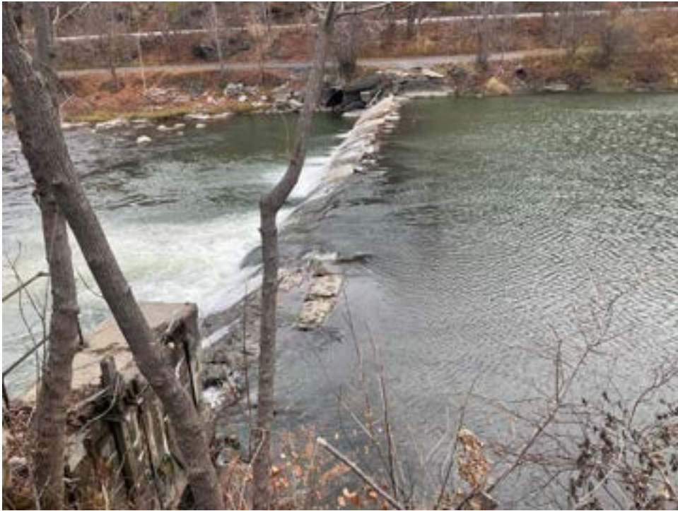
Photo 32. View of Pioneer Dam from the south bank of the Winooski River, facing north.
