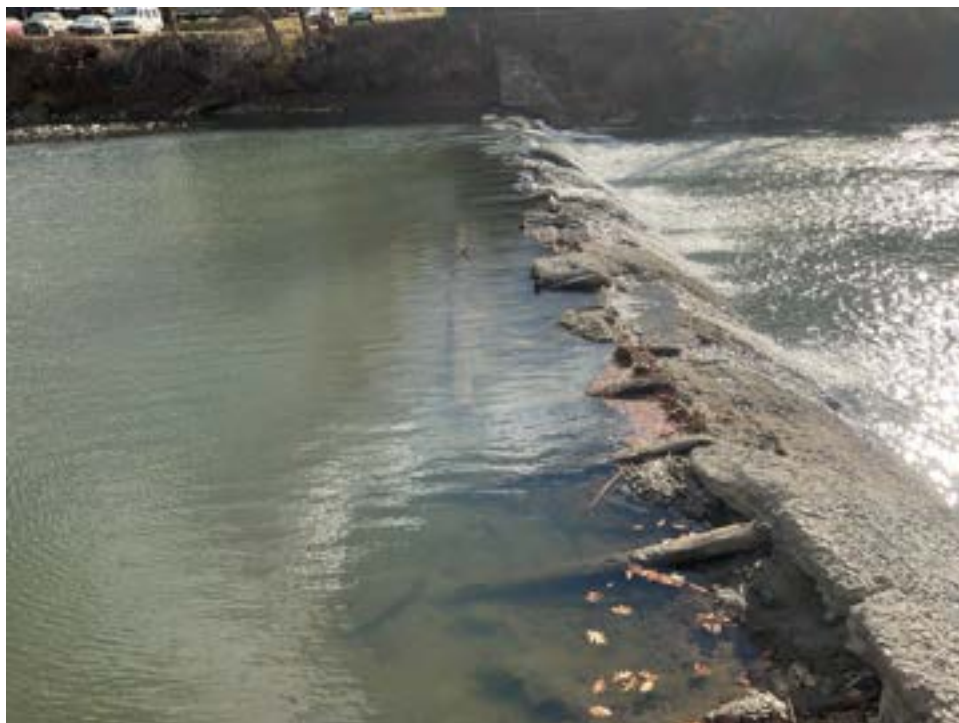
Figure 8. View of Pioneer Dam and former crib dam elements from Old Country Club Road (VHB 2024).
