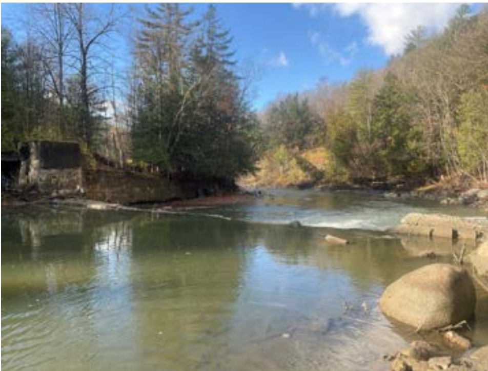
Photo 9. View of Hidden Dam from upstream, facing west.
