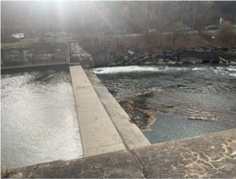
Photo 40. View of the Bailey Dam and stone embankment walls from the former Pioneer Mills, facing southwest.
