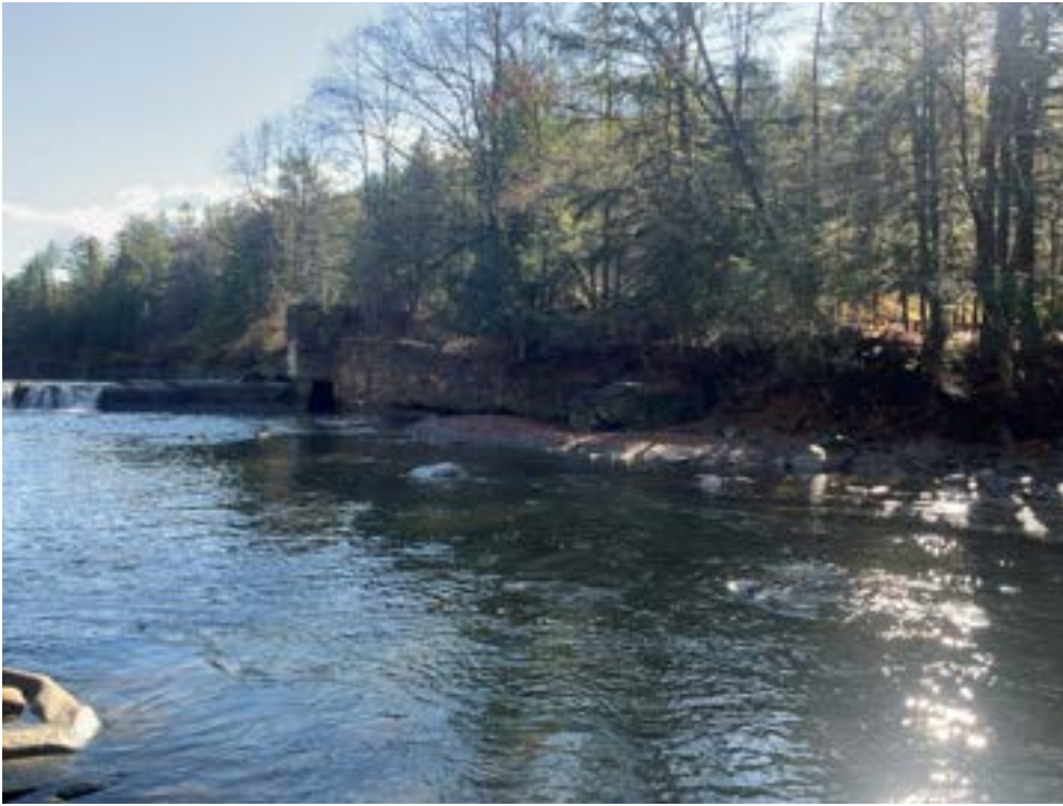
Photo 4. View of Hidden Dam, facing northeast.
