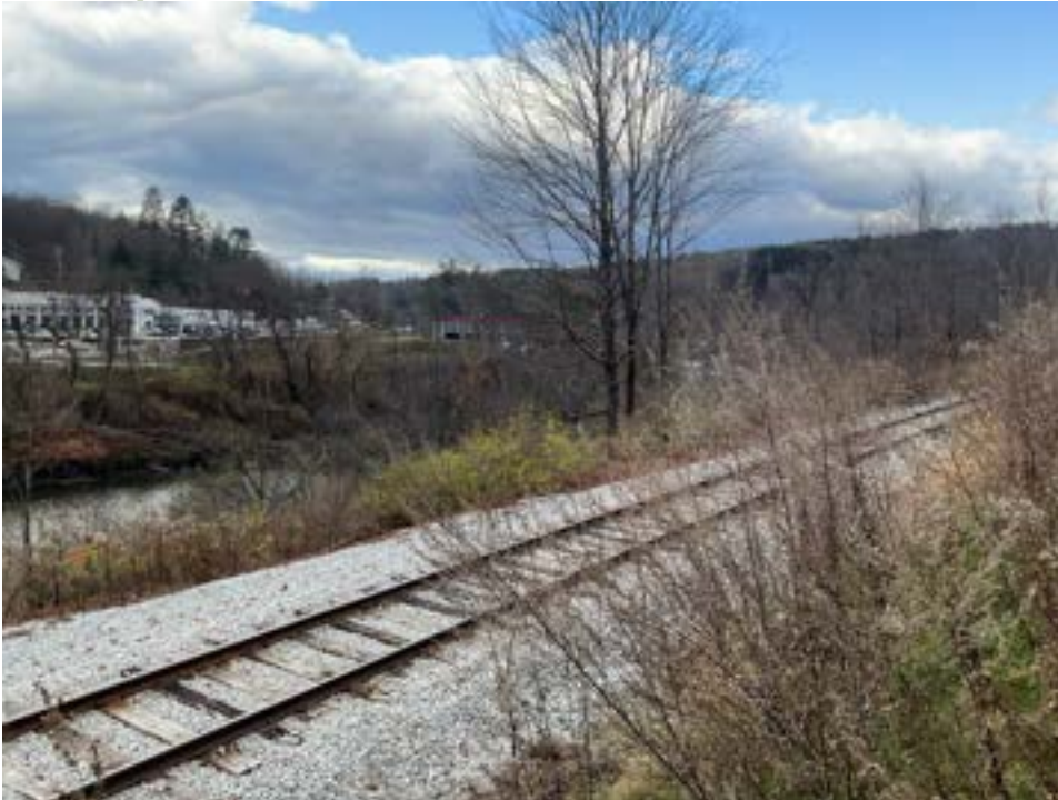
Photo 23. View of railway and Winooski Riverbank, facing northwest.
