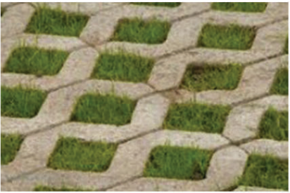
Samples of permeable pavement types: interlocking pavers, spaced pavers and pavers with large voids for grass or gravel
