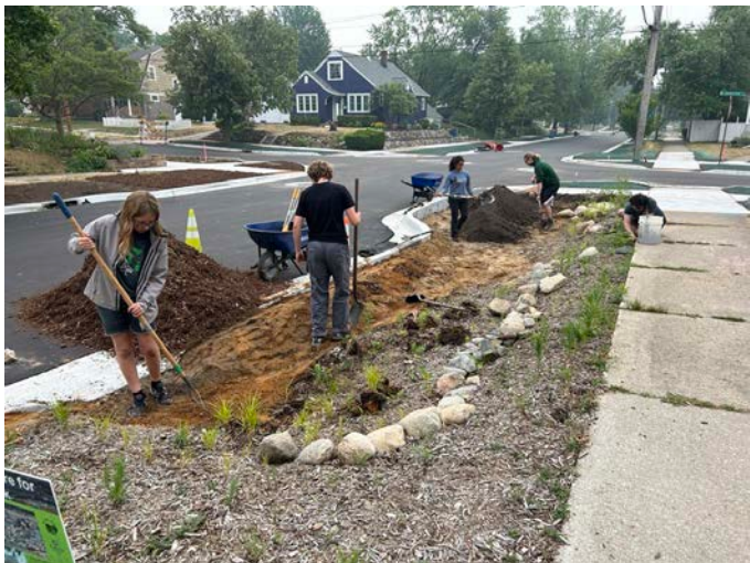
A rain garden installation
