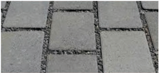
Samples of permeable pavement types: interlocking pavers, spaced pavers and pavers with large voids for grass or gravel
