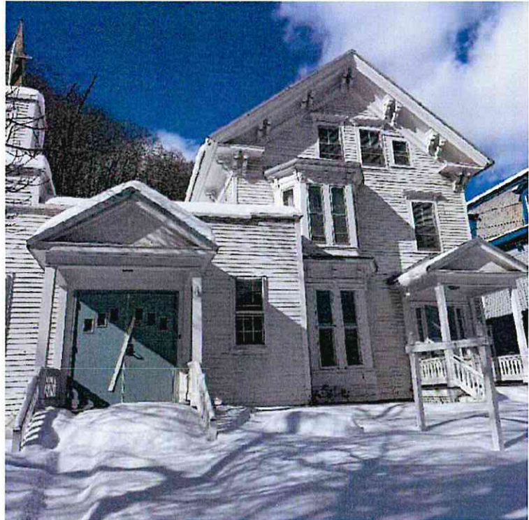
Front (south side) of the building taken from the sidewalk
