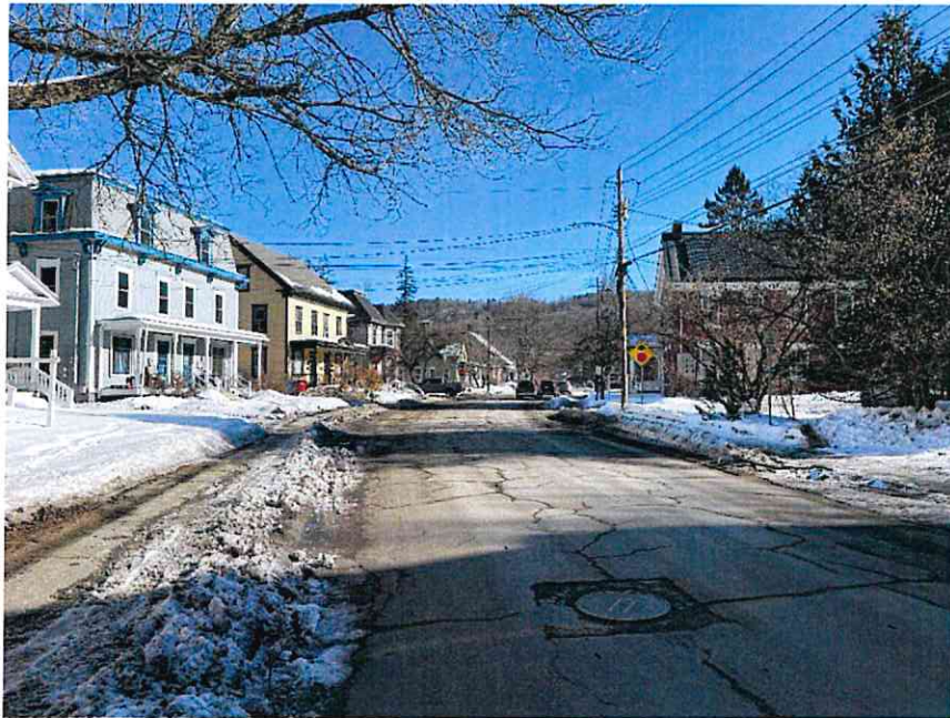
Elm Street Looking North
