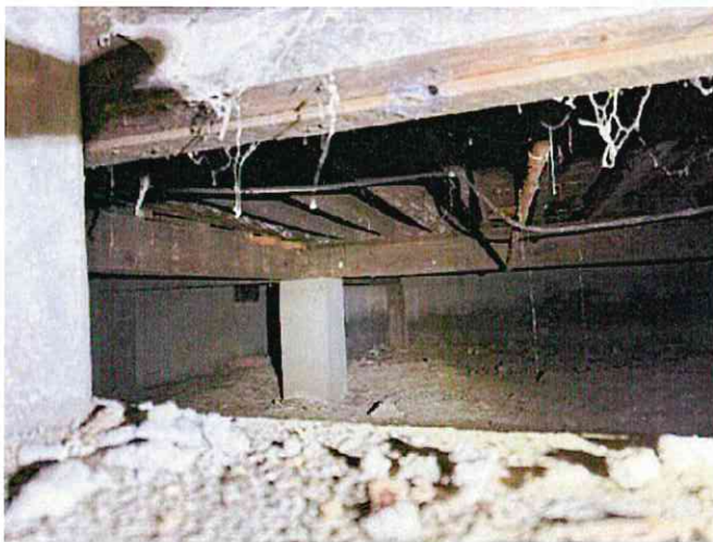
Crawlspace below church hall showing newer foundations with older rough sawn floor framing and plank sheathing
