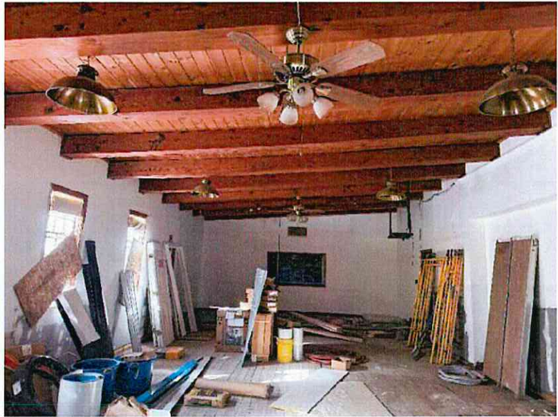
Church hall, recent renovations started, framing mostly concealed
