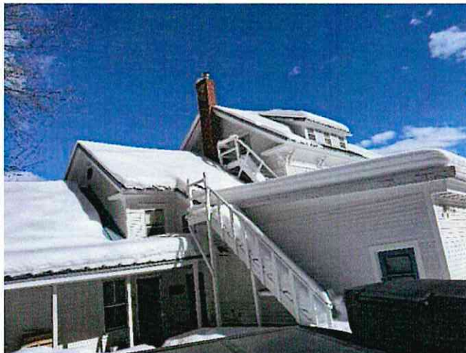
Building from exterior, Northwest corner
