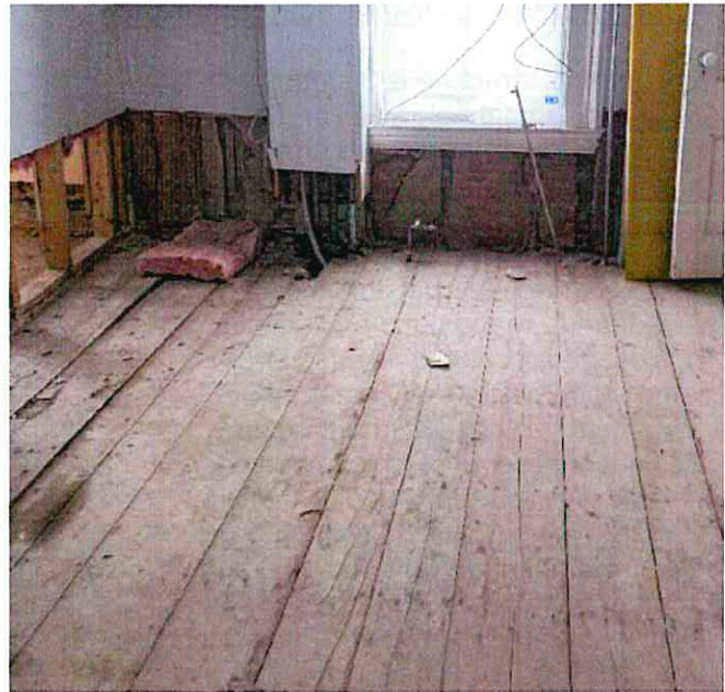
First floor lifting at the interior wall (see left of photo)
