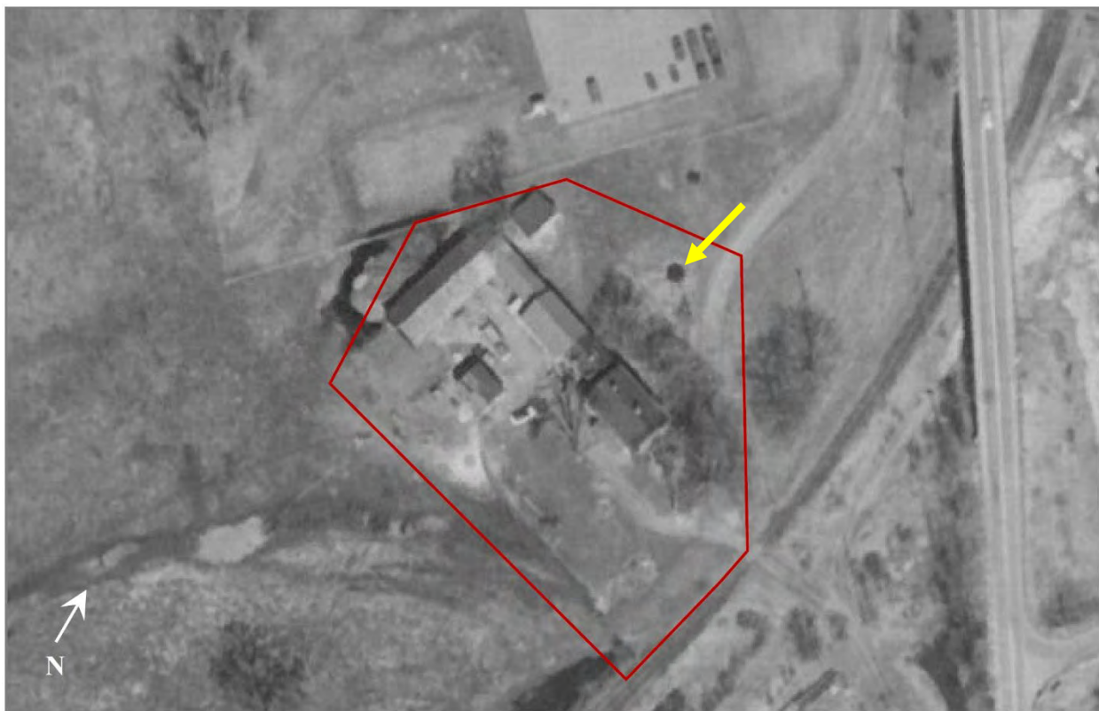
Figure 11. 1969 aerial view of the Jacob Davis House Demolition/Winooski Floodplain Restoration Project, Montpelier, Washington County, Vermont. The yellow arrow points to a small pond or similar water feature possible located near Transect 1.
