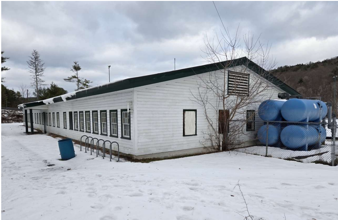
Figure 17. Bathhouse, Recreation Field, Montpelier, VT Date: 2025 Credit: Bob McCullough
