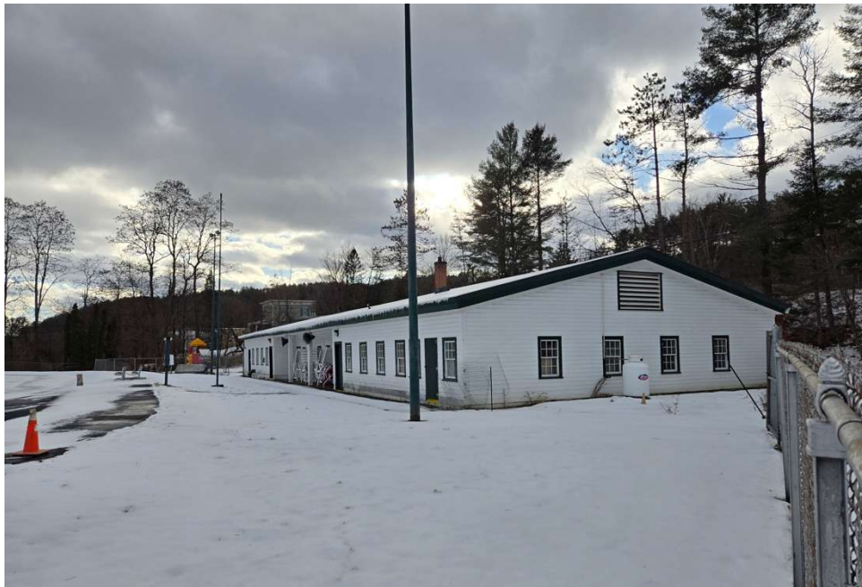
Figure 18. Bathhouse, Recreation Field, Montpelier, VT Date: 2025 Credit: Bob McCullough
