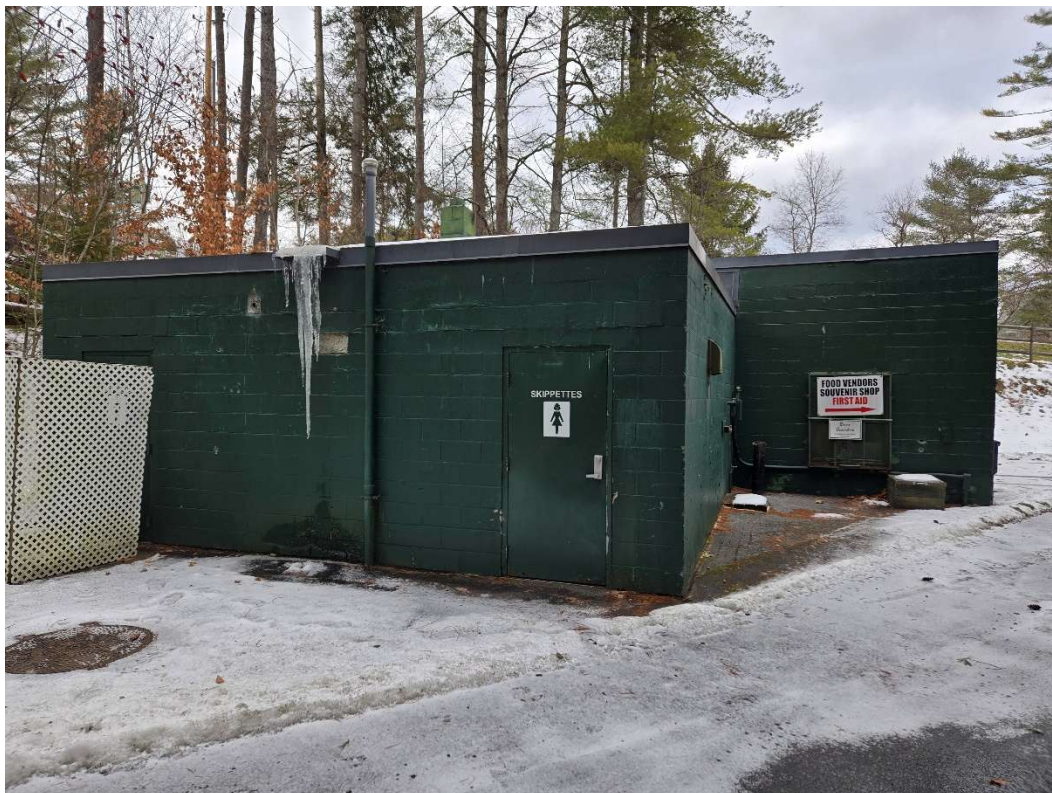
Figure 12. Maintenance Garage and Public Toilets, Recreation Field, Montpelier, VT
