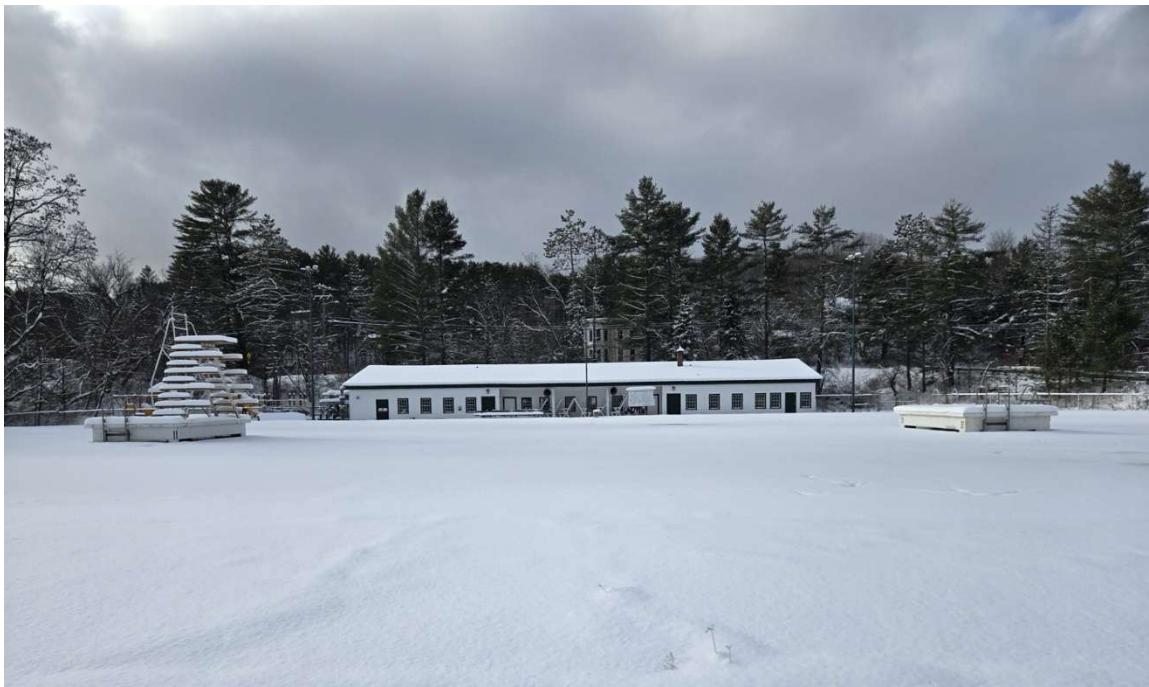
Figure 16. Bathhouse, Recreation Field, Montpelier, VT Date: 2025 Credit: Bob McCullough
