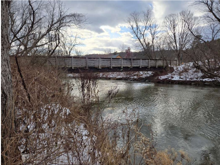
Figure 21. Pedestrian Bridge, Recreation Field, Montpelier, VT Date: 2025 Credit: Bob McCullough
