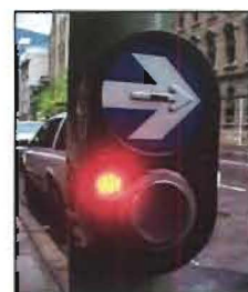
Example of accessible pushbutton with raised arrow and large diameter
