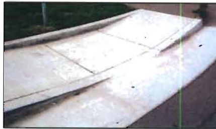
Correct way to provide ramp on narrow walks.
