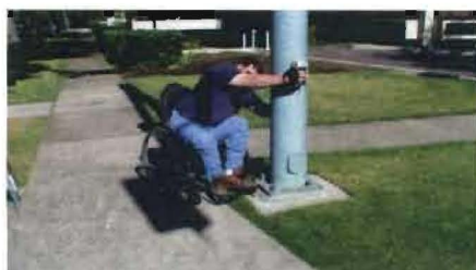
Button not accessible from sidewalk
