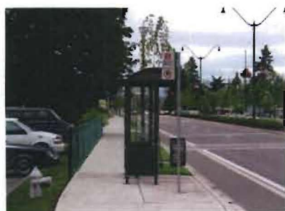
Bus shelter accessible from sidewalk
