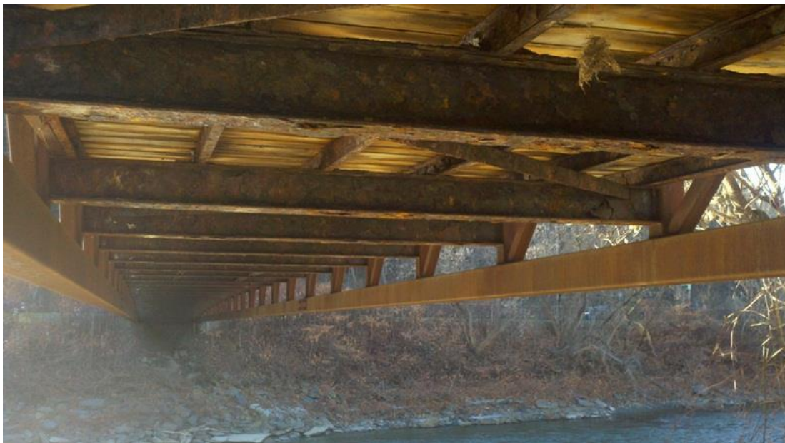
Figure 2 Underside of Pedestrian Bridge
