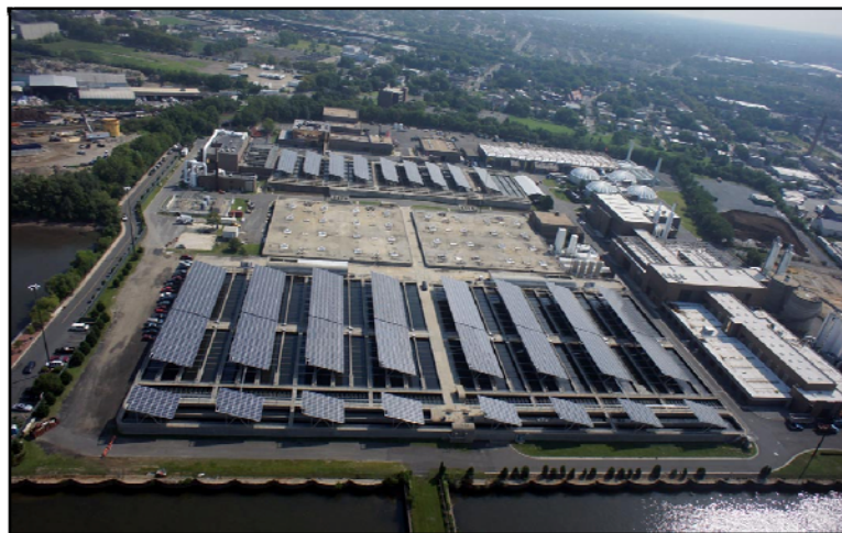
GRO SOLAR'S 1.8 MW CAMDEN COUNTY MUNICIPAL UTILITY AUTHORITY PROJECT
