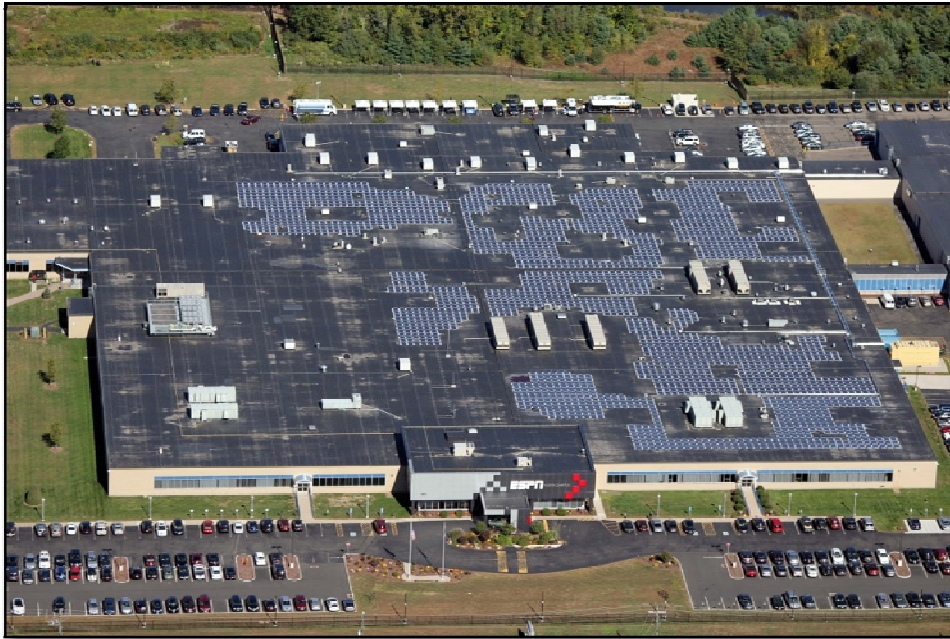
GROSOLAR'S 663 KW ESPN HQ PROJECT
