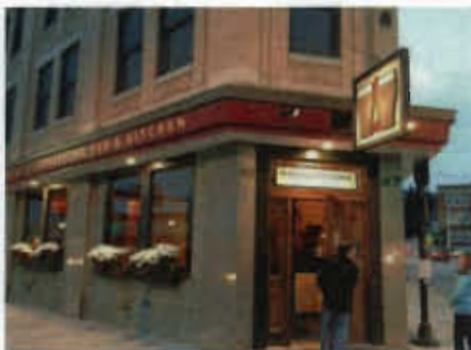
Cornerstone Pub and Kitchen, with offices and apartments above it, Barre, VT
