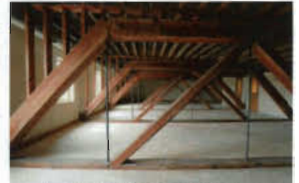
Blanchard Block attic renovate for office use
