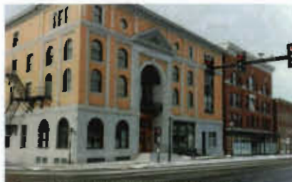
Barre City Hall Exterior Restoration
