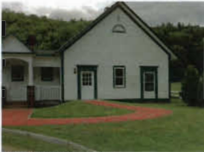
Granville Municipal Offices
