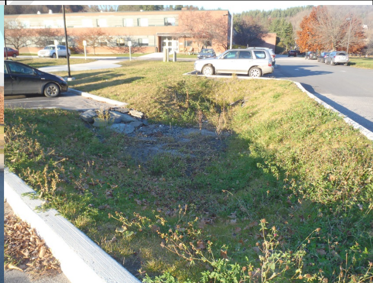
Photo 2. Existing stormwater management in back parking lot
