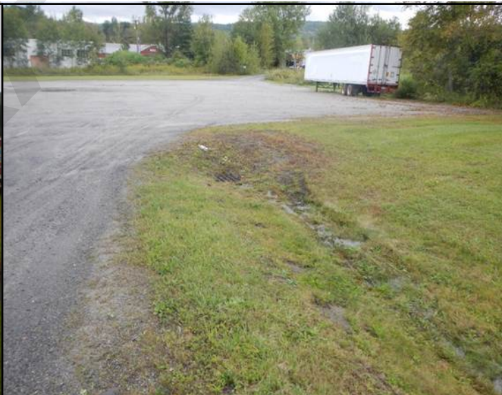
Photo 2. Ditch that could be reshaped and stabilized to provide better treatment for storm water before it reaches the pond.
