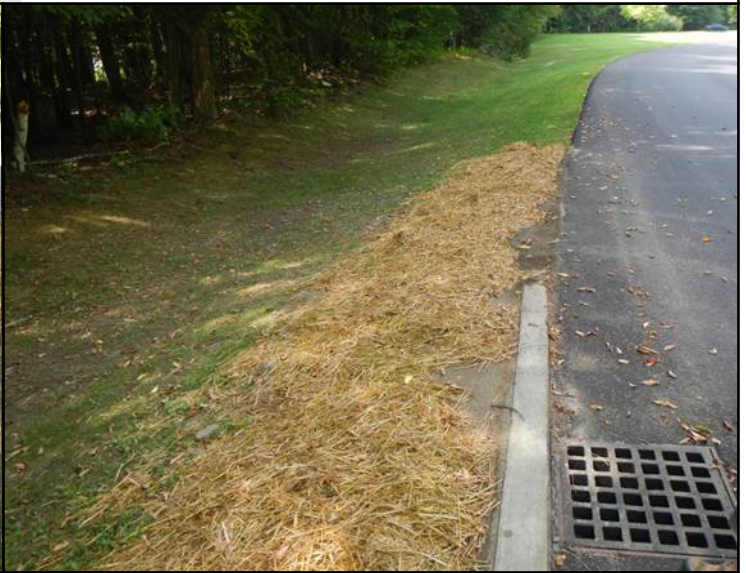
Photo 2. Catch basin uphill of green space
