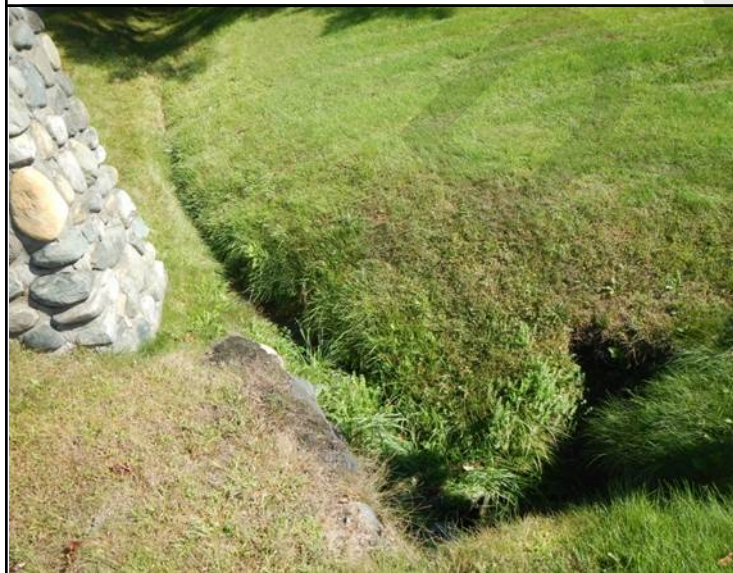
Photo 1. Narrow ditch that needs to be expanded.
