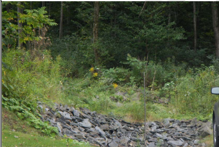
Photo 1. Rock pile constructed in the yard of the topmost house in the line of flow
