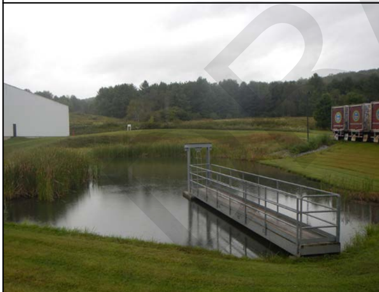
Photo 1. Pond between the two building complexes
