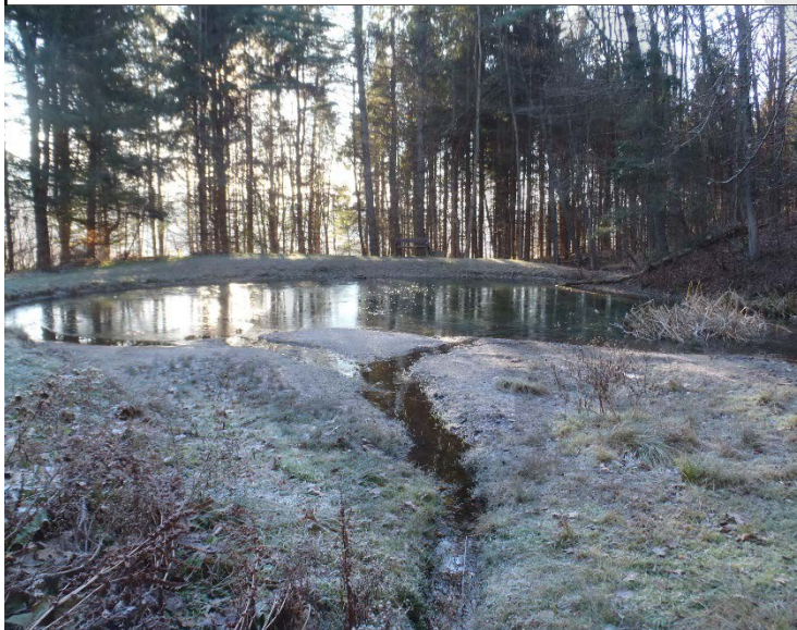
Photo 1. Sediment accumulation at pond inlet
