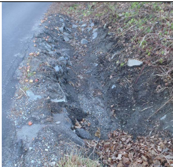
Photo 2. Sediment accumulation in drainage ditch
