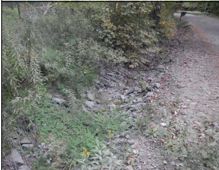
Photo 1. Rock-lined ditch in need of improvement.
