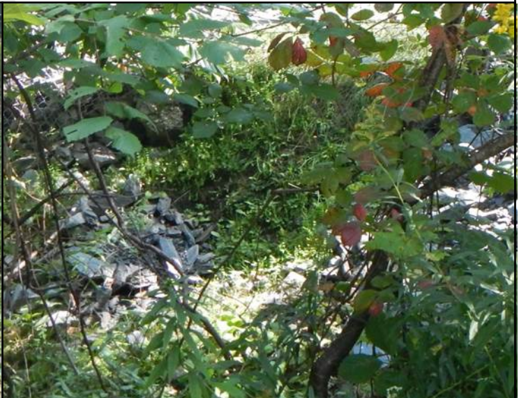
Photo 2. Pipe outlet across the fence
