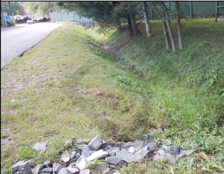
Photo 1. View of swale behind parking lot
