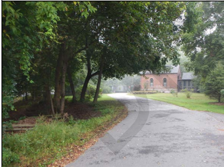
Photo 1. View of Arsenal Drive toward College St. Hill slope is to the left of this photo.
