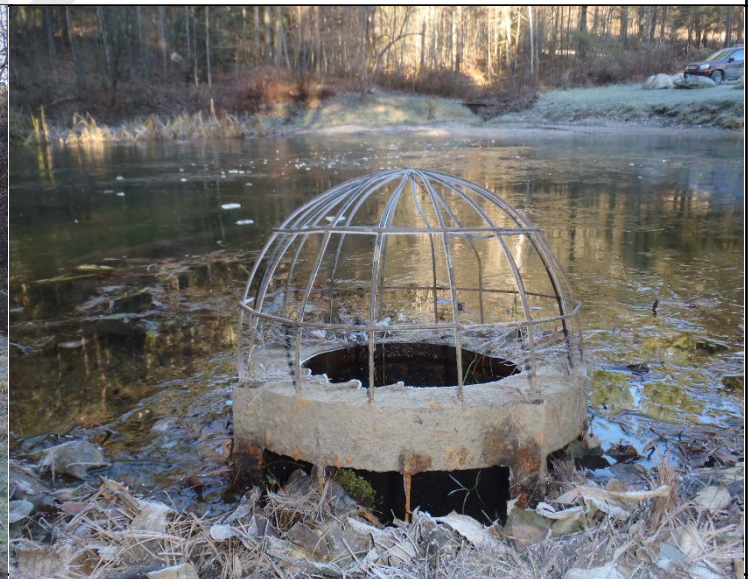
Photo 2. Existing pond outlet structure
