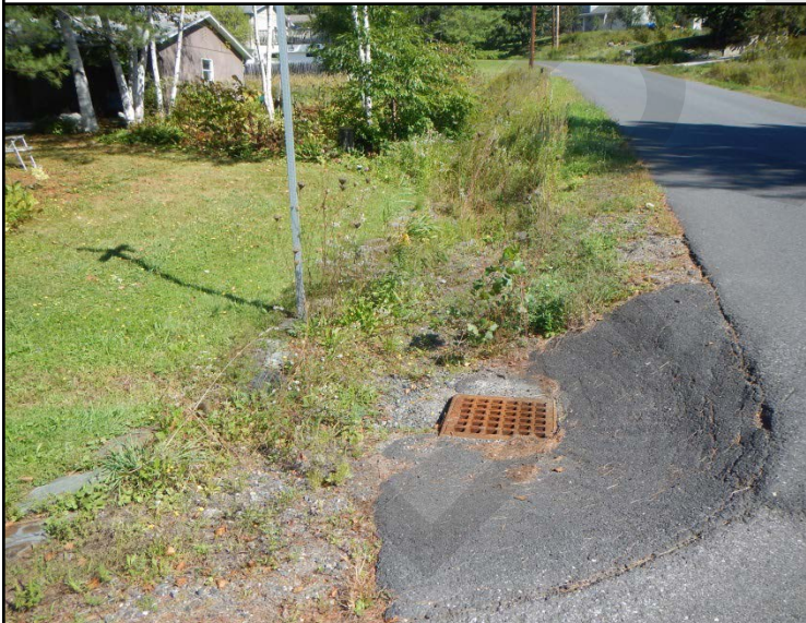
Photo 1. Catch basin and potential treatment area.
