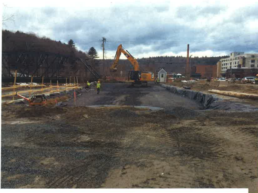
On-going placement of granular material
