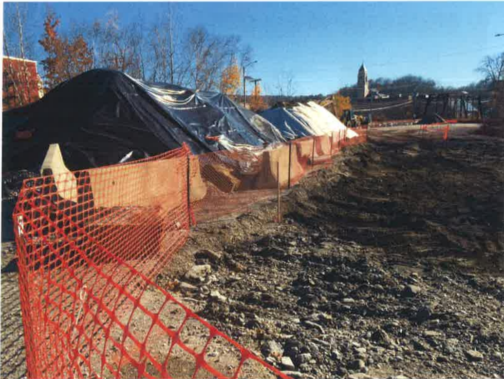
Soil stockpiles: Note fully encapsulated in barrier per CAP
