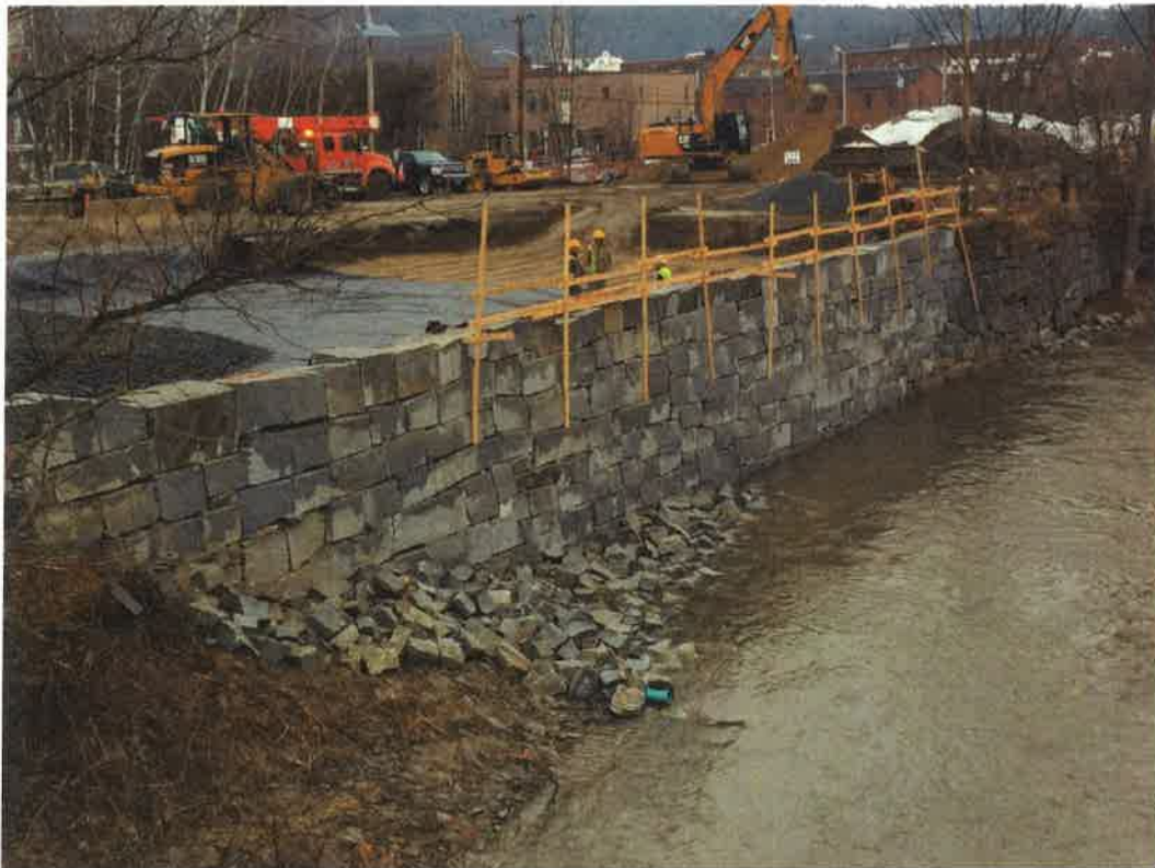
Near final completion of wall: March 2017
