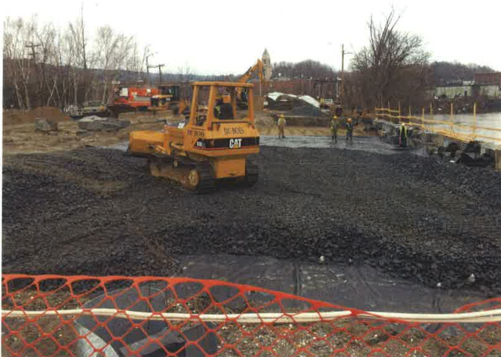
Placement of granular material behind wall: March 2017
