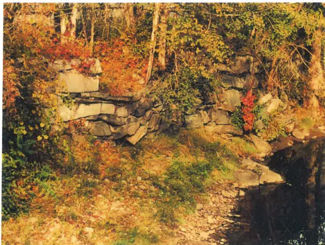
Close-up of failed wall section Pre-construction: Sept 2016
