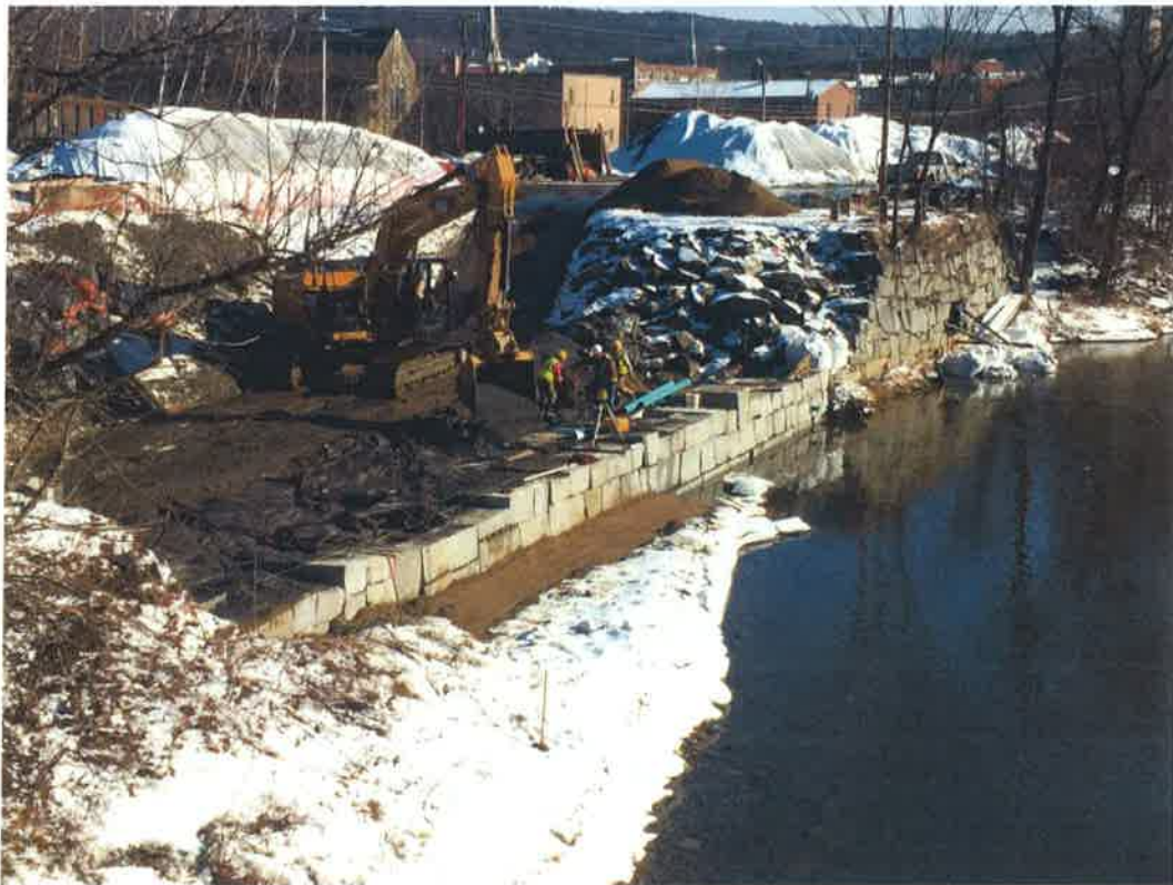
The wall begins to take shape: Feb 2017
