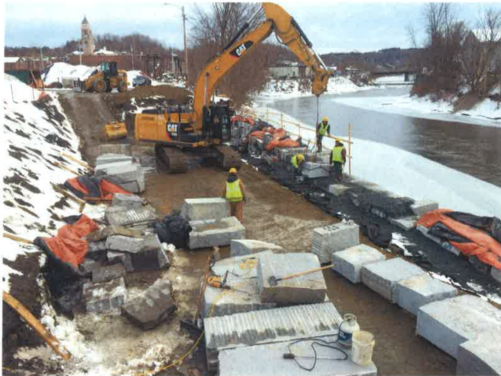
Placement of granite blocks, individually set into place: Feb 2017
