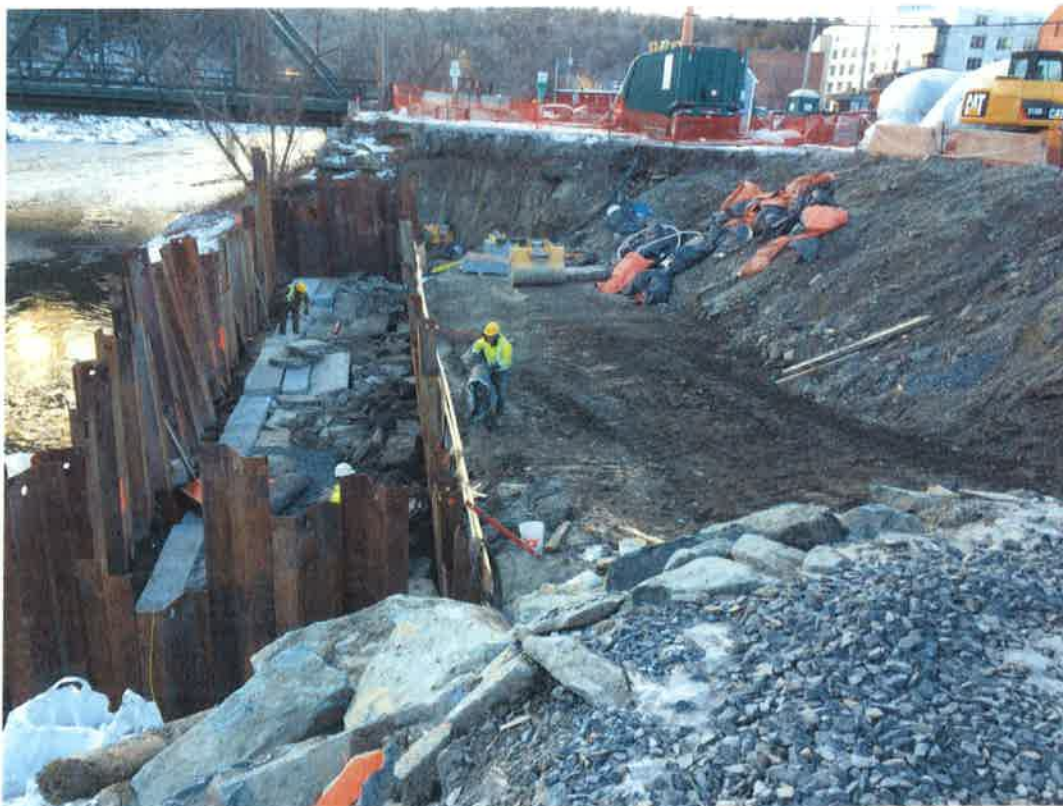
Initial placement of granite block wall on top of concrete foundation: Jan 2017
