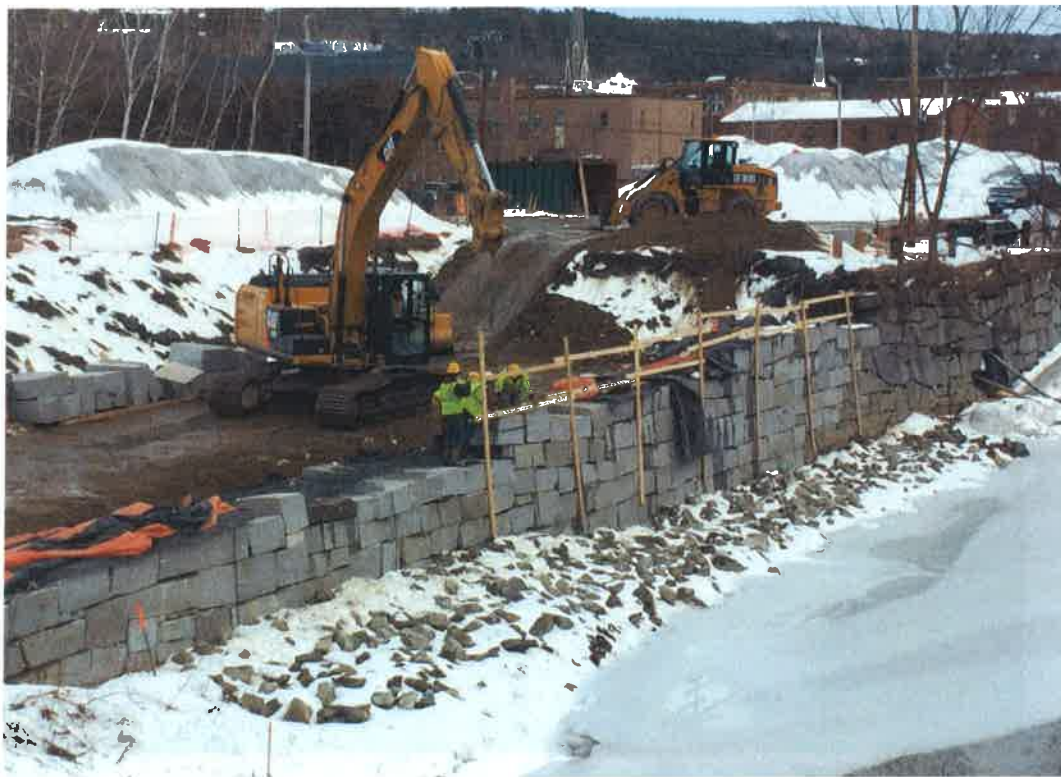
Wall nears half-way up: Feb 2017
