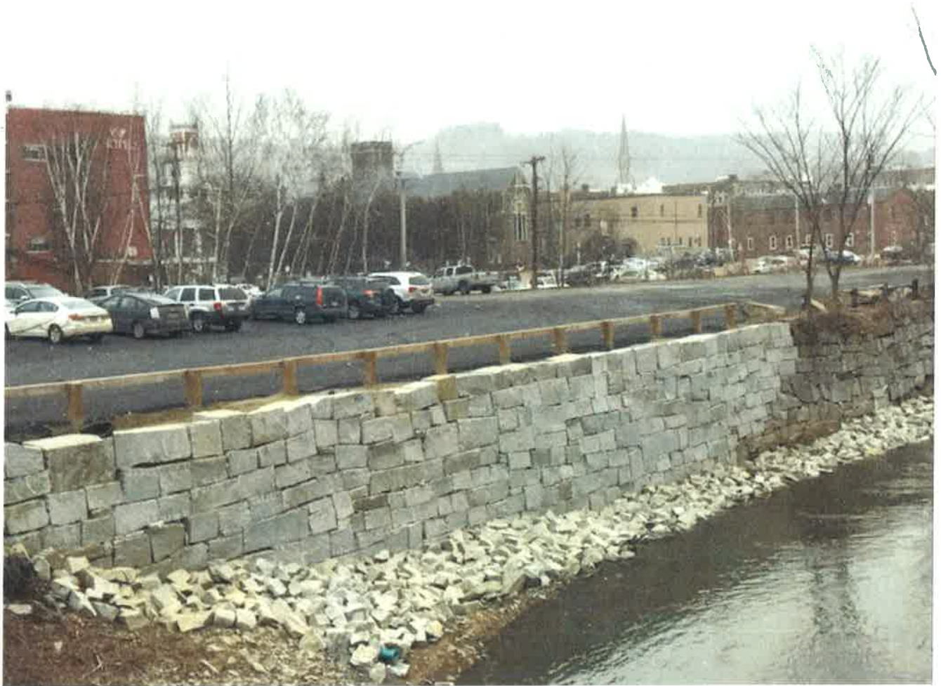
Final completion: April 2017
