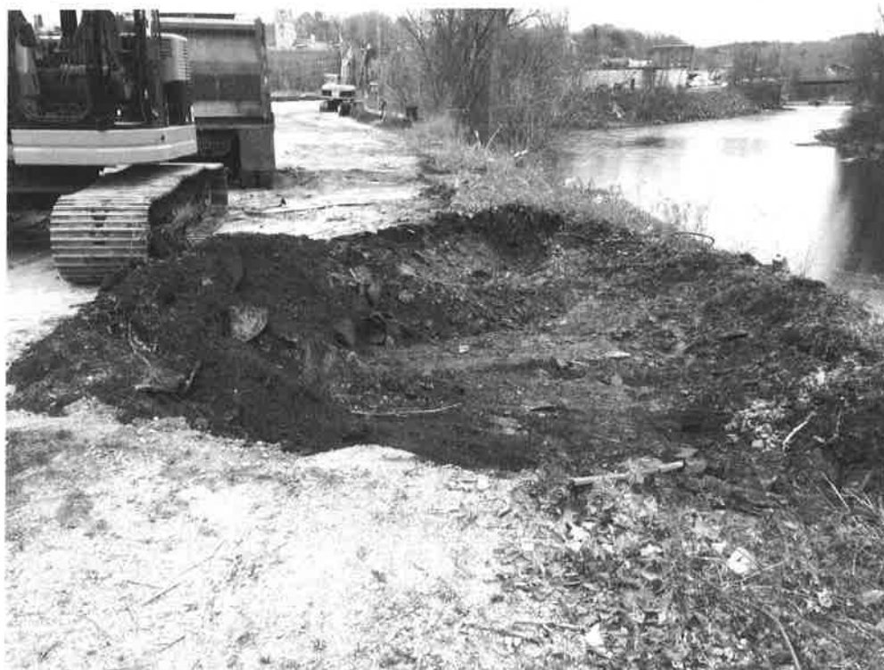
Initial excavation behind wall: Nov 2016
