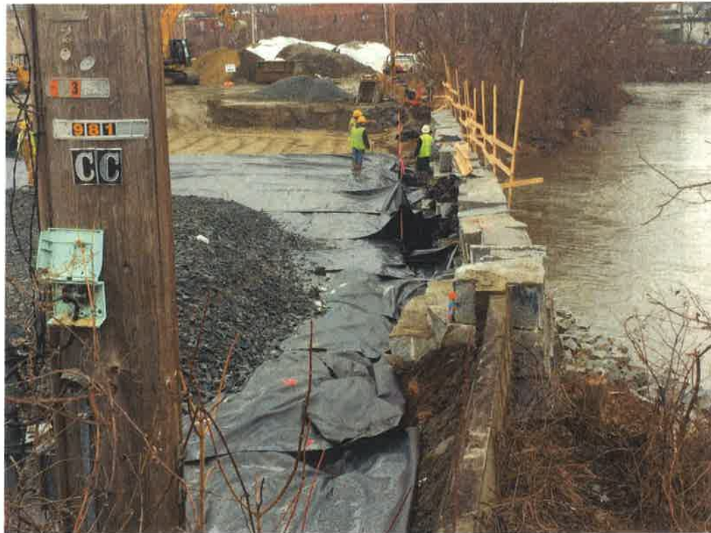
Close-up of backfill behind near completed wall: March 2017
