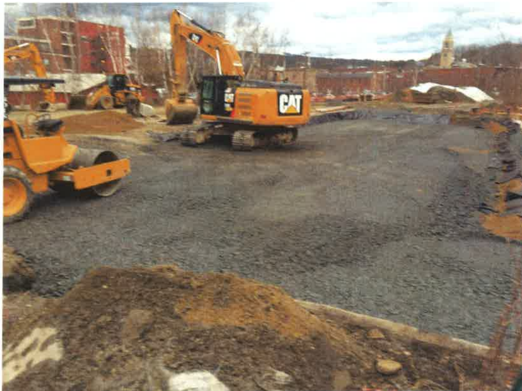
Placement and compaction of granular material: March 2017
