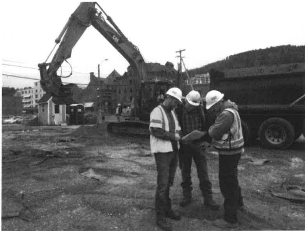
Engineers & contractor review plans on first day of excavation: Nov 2, 2016
