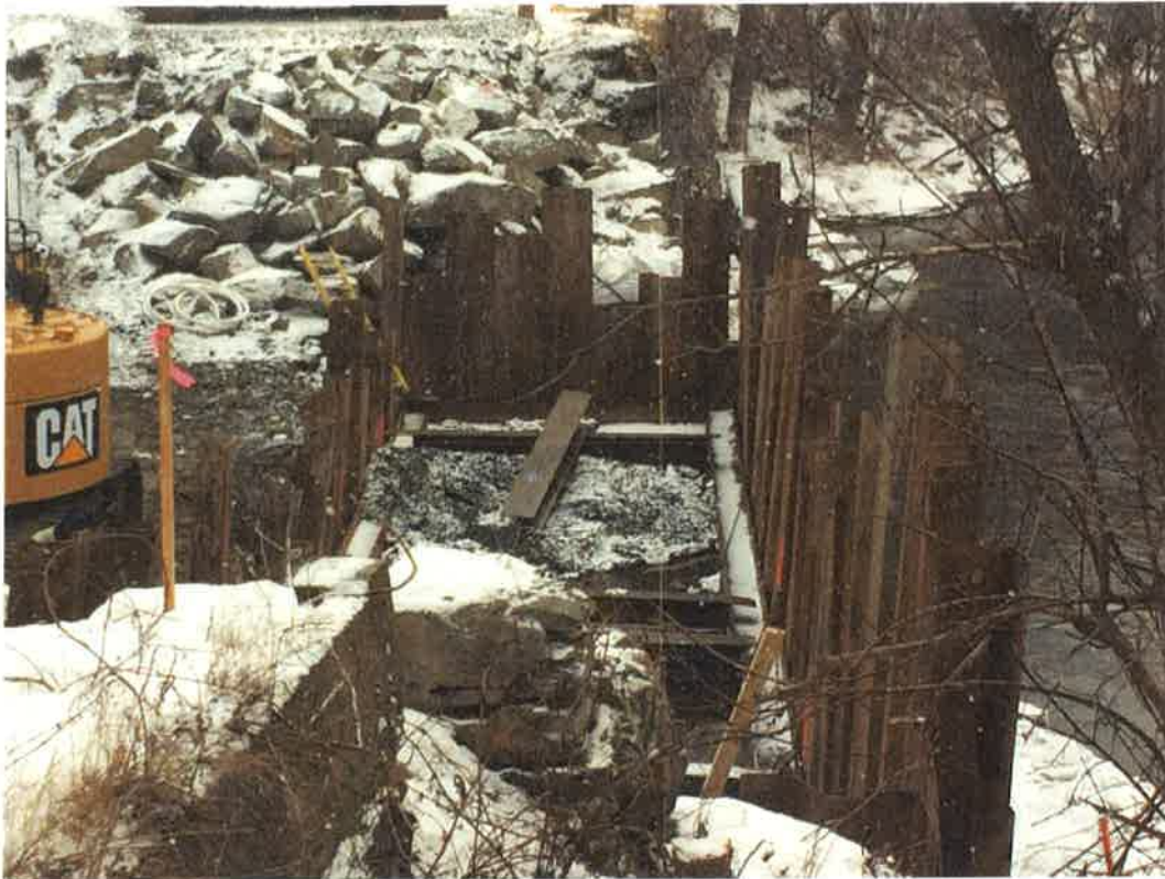
Wall foundation excavation, note sheet piling isolates work from river: Dec 2016
