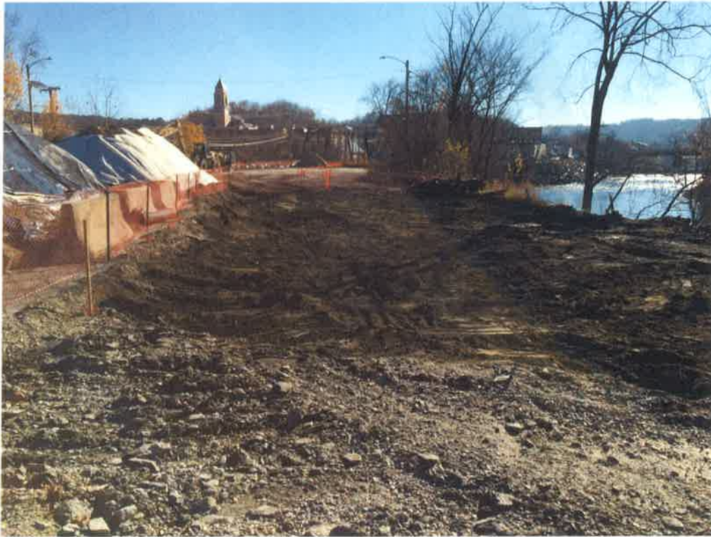
On-going excavation: Note soil stockpile to left
