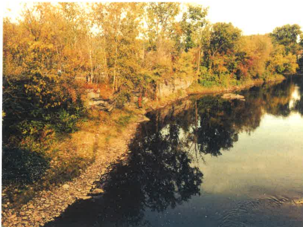
Pre-construction condition of wall: Sept 2016
