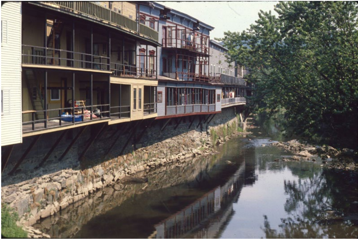
Figure 8: Late-1970s photograph by Courtney Fisher of the rear of the three buildings along the North Branch.
