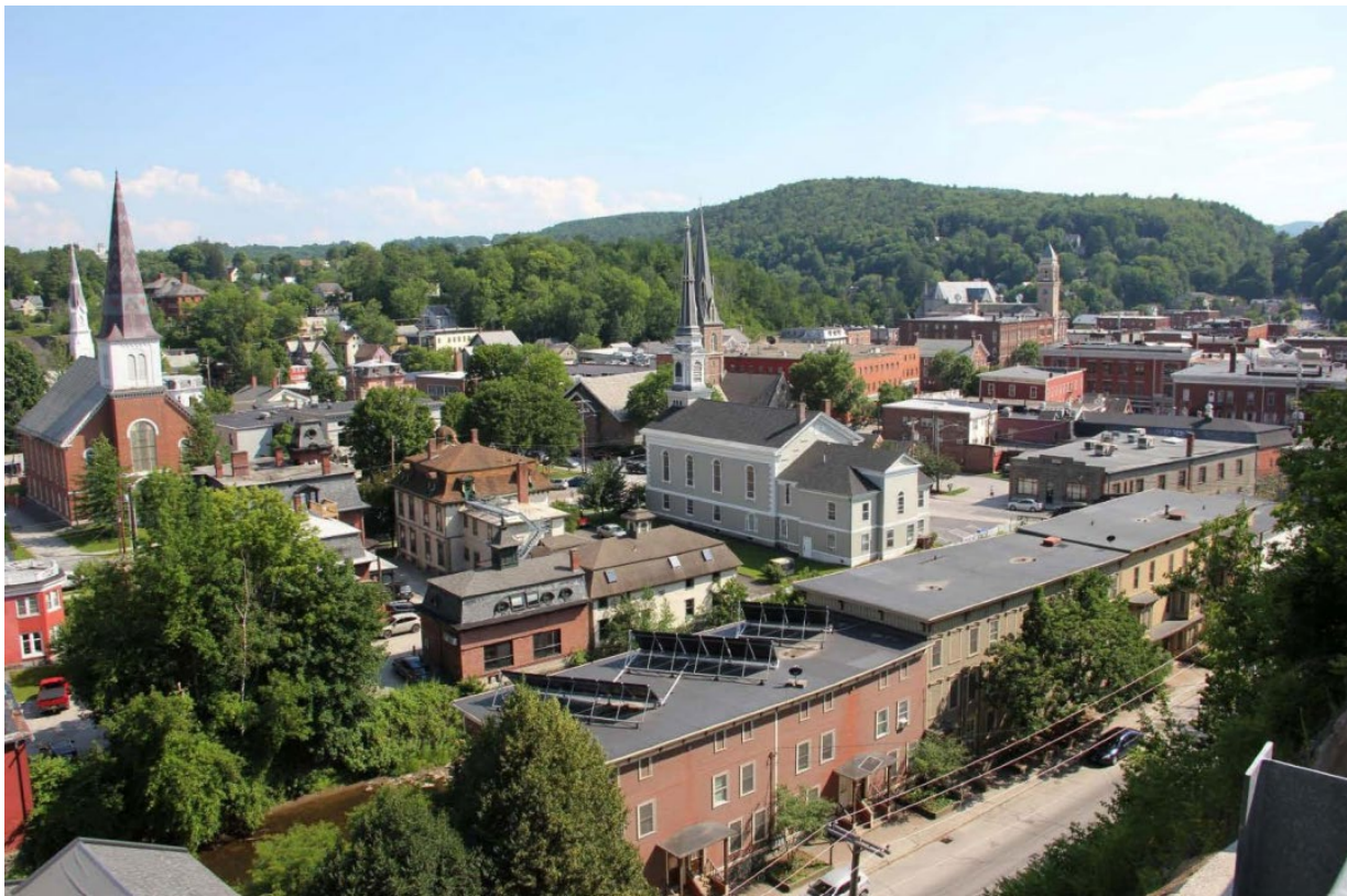
Figure 10: 2016 photograph of the buildings, looking south, by Lyssa Papazian for the National Register nomination update.
