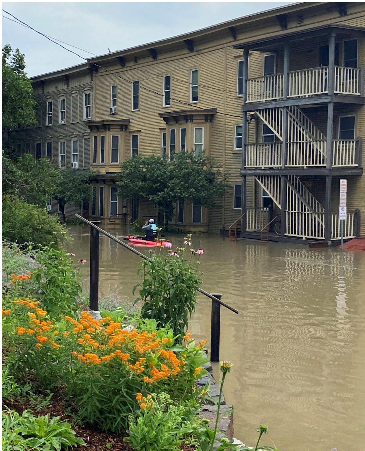
Figure 11: Photograph of the building during the July 2023 flood.
