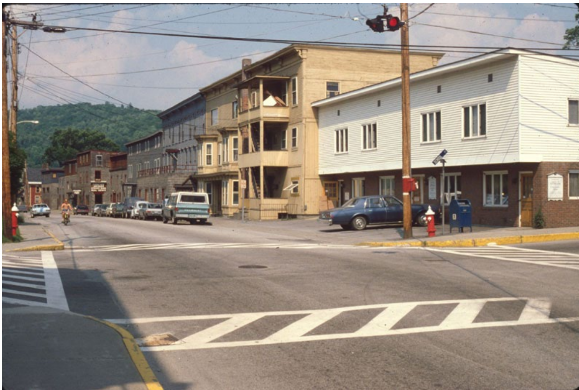
Figure 7: Late-1970s photograph by Courtney Fisher showing the buildings. Note the concrete block addition on Building B's façade at center left.
