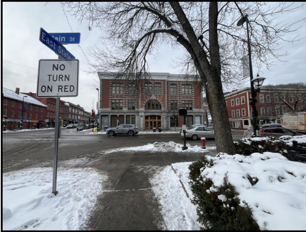
Photograph 27: View of 89 Main Street (location 10) within the Montpelier Historic District.
