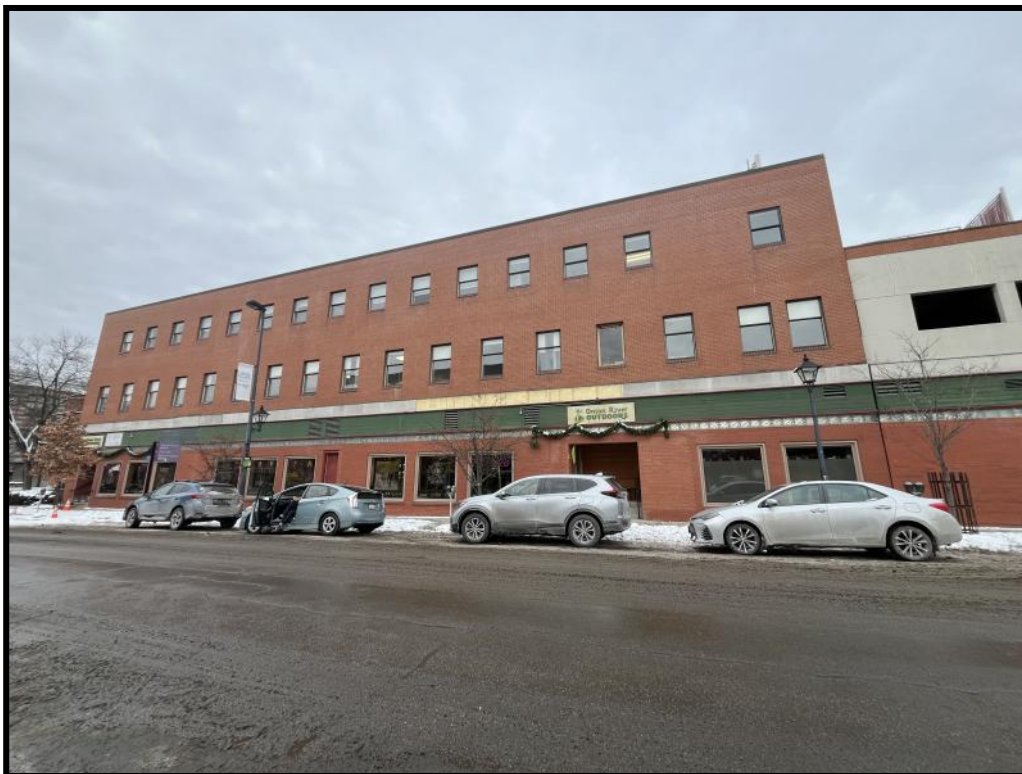
Photograph 10: View towards the site from location 1 (visible).
