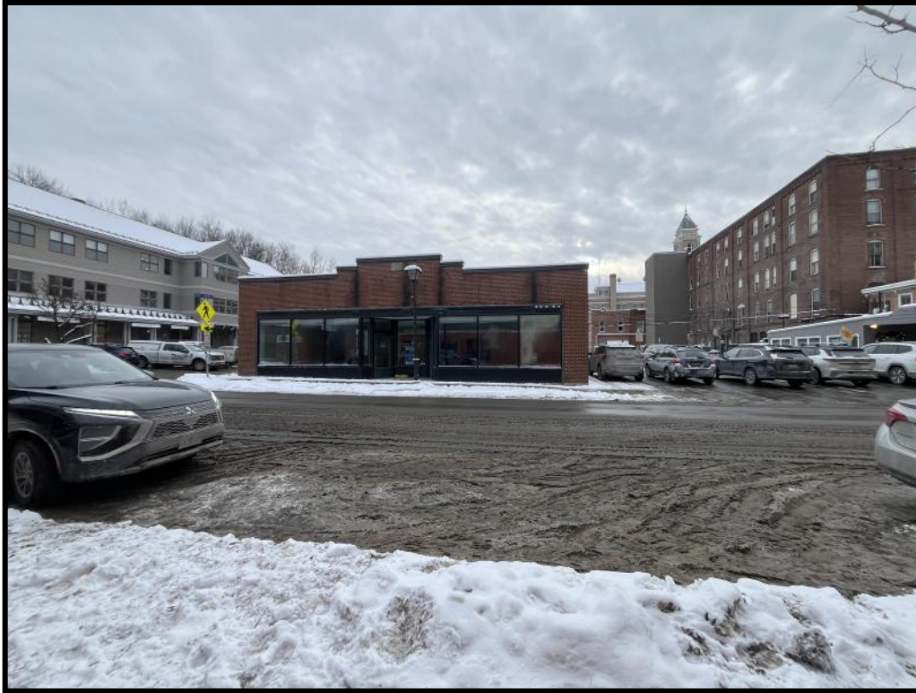
Photograph 9: View of 7 East State Street (location 1) within the Montpelier Historic District .
