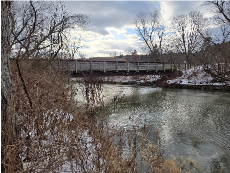
Figure 20. Pedestrian Bridge, Recreation Field, Montpelier, VT
