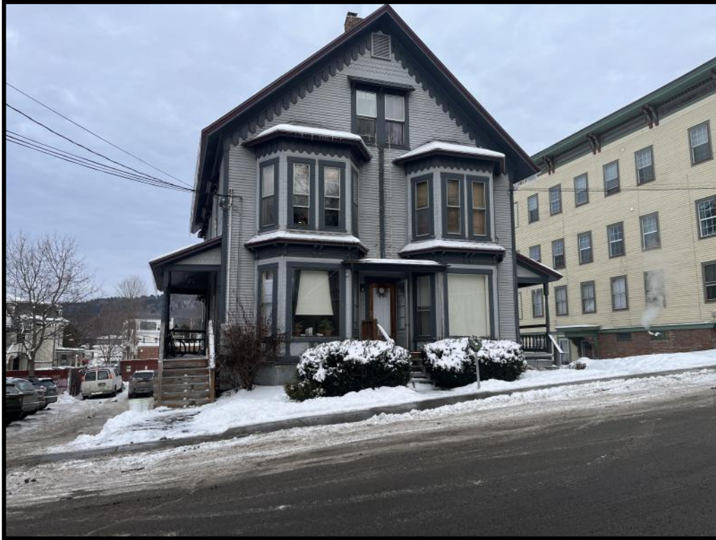
Photograph 15: View of 32 East State Street (location 4) within the Montpelier Historic District.
