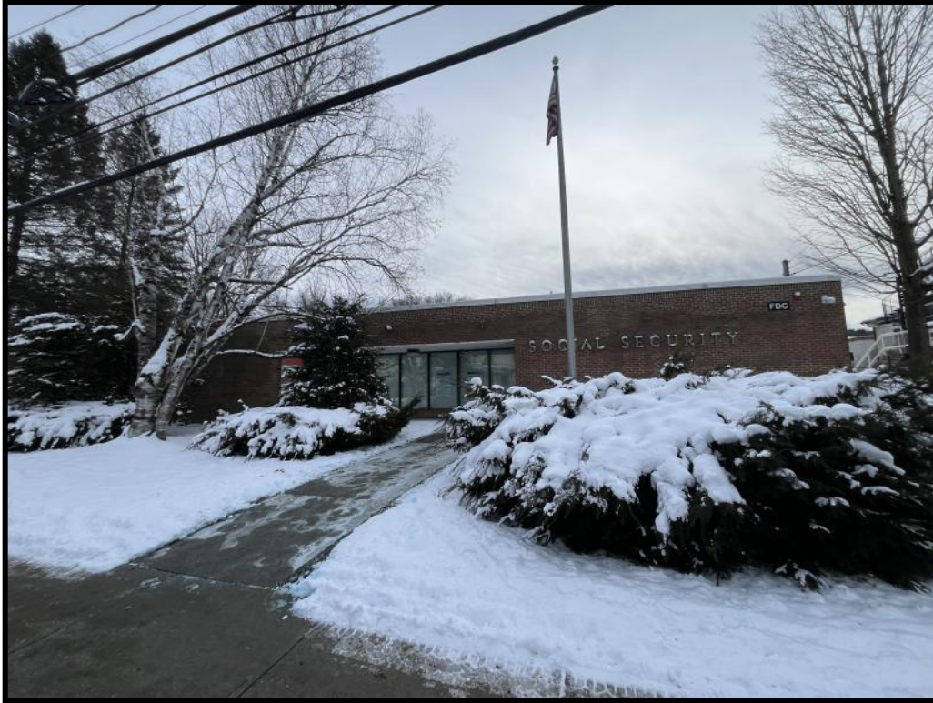
Photograph 17: View of 32 School Street (location 5) within the Montpelier Historic District.
