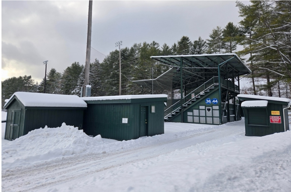
Figure 11. Grandstand, Ticket Booth, and Concession and Souvenir Stand, Recreation Field, Montpelier, VT
