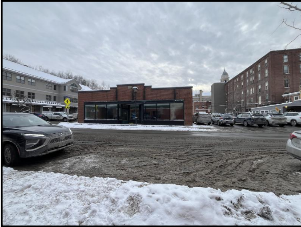
Photograph 11: View of 11 East State Street (location 2) within the Montpelier Historic District.
