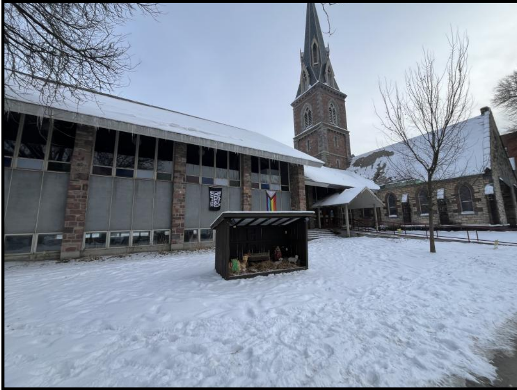
Photograph 21: View of 26 School Street (location 7) within the Montpelier Historic District.
