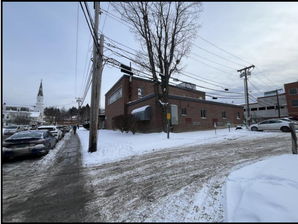
Photograph 19: View of 23 School Street (location 6) within the Montpelier Historic District.
