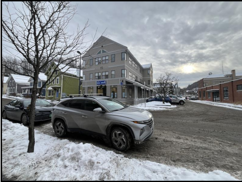
Photograph 13: View of 15 East State Street (location 3) within the Montpelier Historic District.
